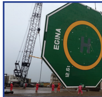
■ Helideck and support ready for loadout
